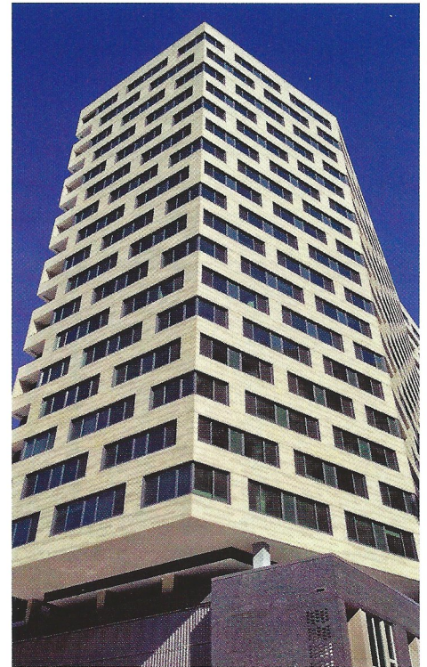
The west (right) and south elevations of Eleven55 Ripley luxury apartments shine in February afternoon sunlight. Beneath the clay masonry exterior, the building relies on two separate air barrier systems. Photo courtesy of Jim Glaze, Thomco Inc.
