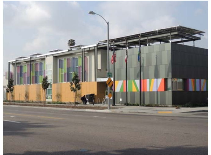
Over 4,300 sq. ft. of Wrapshield Water Resistive Vapor Permeable Air Barrier Membrane was installed under Trespa panels.
